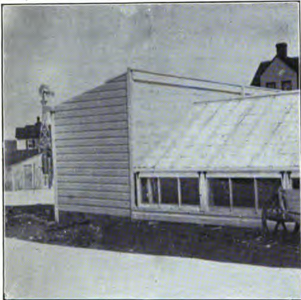
10.—Shed at north end of houses, showing method of construction. Shed has glass roof.
